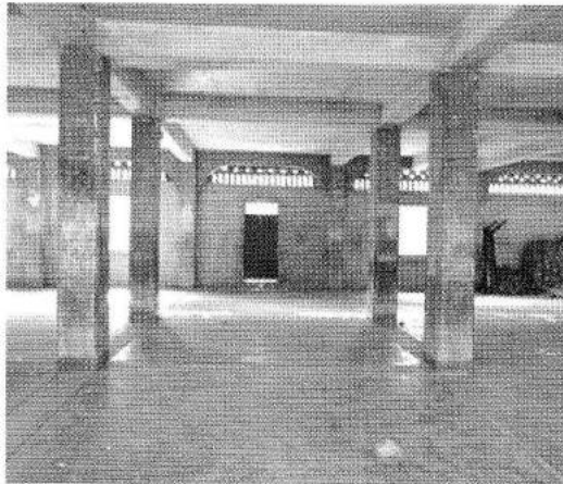
Plate-1 (Soft Storey) Location- Lombpri Para Govt Primary School N-21°25' 05.750 " ; E-92°05' 36.913 " Union: Chakmarkul
